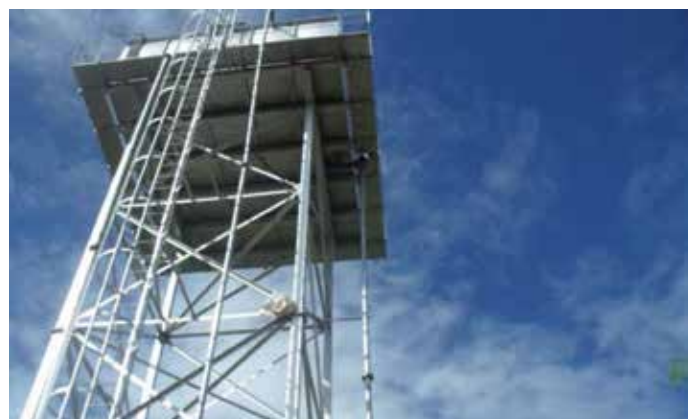
50,000 Litres water reservoir constructed at Migyera
